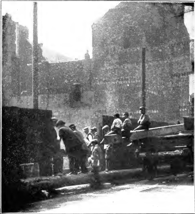
Boys who have left their youthful pursuits to watch the construction of a building
